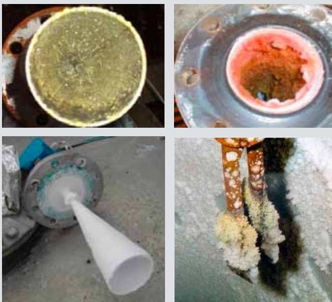
Fig. 5: Examples of sensor connections affected by the process
